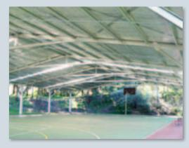
Safety and security under cover are also important. Ranbuild have removed the potentially dangerous diagonal wall braces and replaced them with lateral braces high up the columns and out of harm's way. Ranbuild COLAs also feature unique 'folded edge' column flashings to reduce the risk of contact with sharp metal edges.
